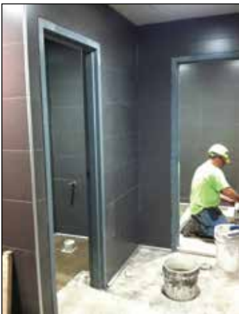
Bathroom during remodeling process
