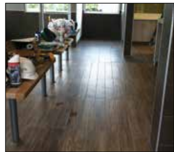
Floors in progress
